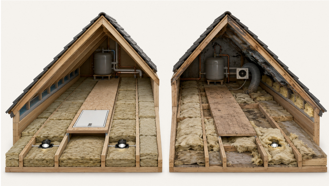
Figure 9 – Coordinated loft insulation compared with common defects.
